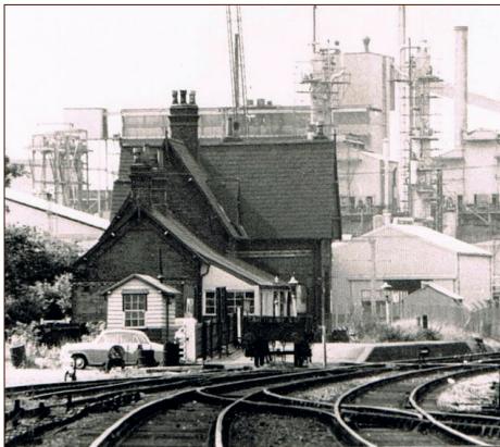
The Lurgi Gas Plant near Coleshill Station
