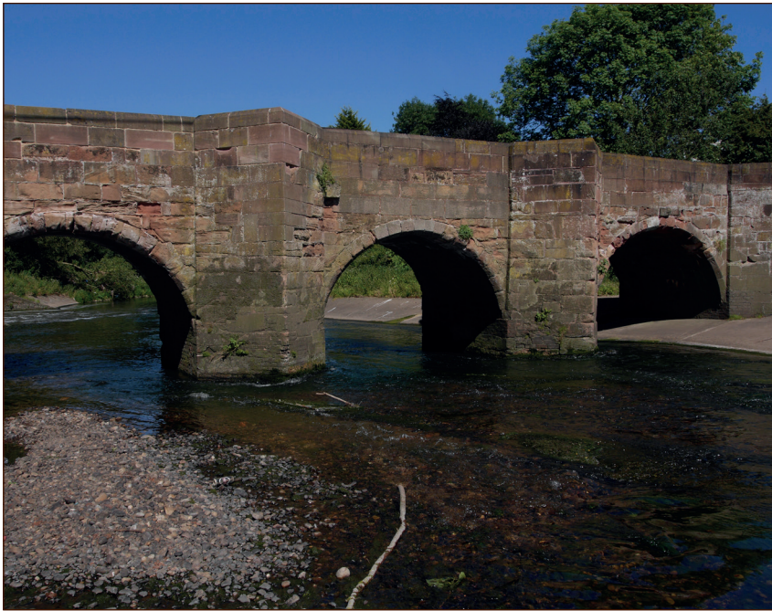
The Tudor bridge at Water Orton
