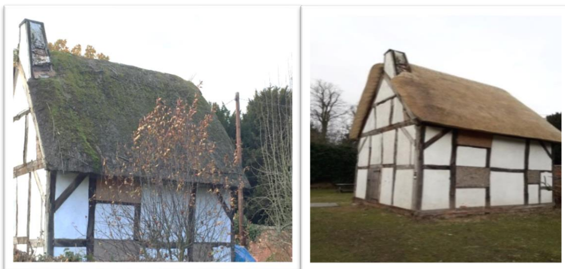
Figure 78: Lea Ford Cottage, before and after replacement of the thatched roof (TVW 2019)
