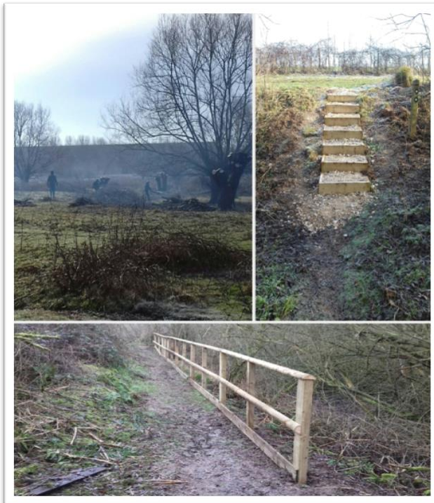
Figure 23: Whitacre Heath tree and access works. Top left: pollarding willow; top right: new steps installed; below: new handrail (E Asbery and TVW 2019)
