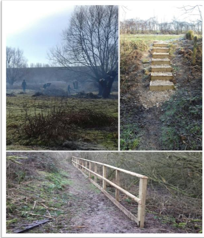
Figure 81: Whitacre Heath tree and access works. Top left: pollarding willow; top right: new steps installed; below: new handrail (E Asbery and TVW 2019)
