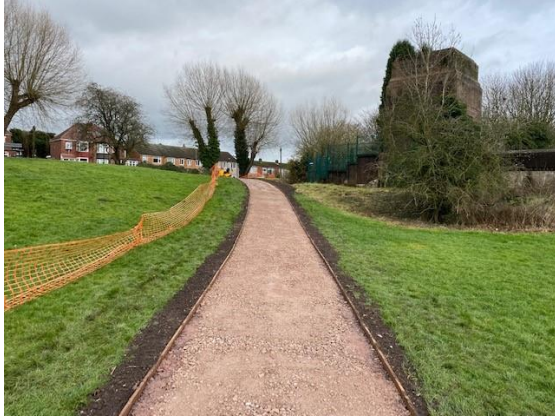
New path in Cole End Park to improve accessibility. Source: NWBC.
