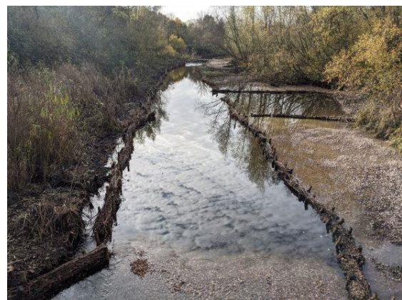
Completed works at Kingshurst Brook. Source: Tame Valley Wetlands
