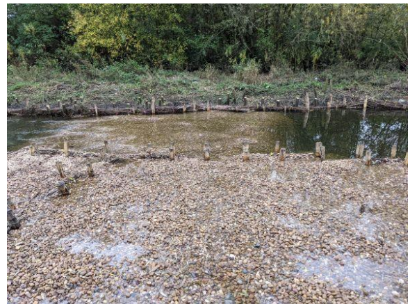
During works, but a section where gravel has been installed, creating riffles. Source: MRE
