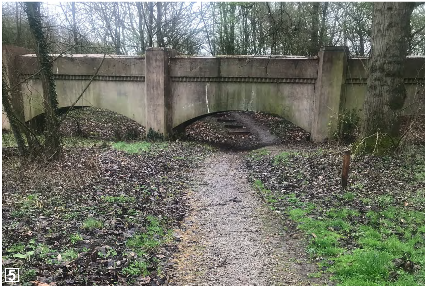
5 Concrete aqueduct / conduit – Arches provide pedestrian permeability but restrict headroom – viewed from the east towards wildlife area.
