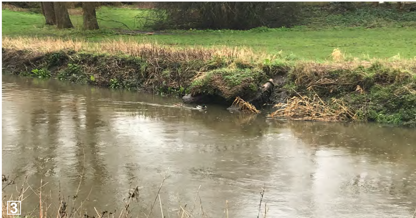
Collapsed culvert on southern bank of river.
