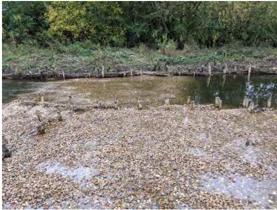
Kingshurst Brook with shingle added. Source: MRE Unlocking Enterprise
