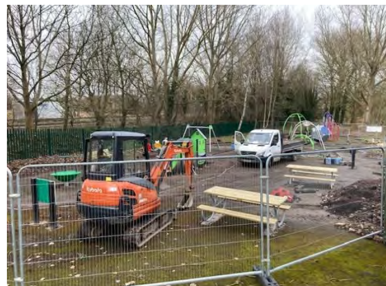
Works for playground underway. Source: NWBC
