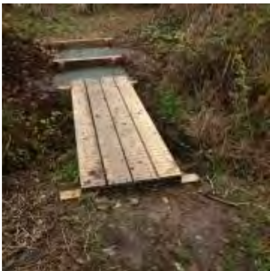
Bridge over ditch/stream. Source: MRE
