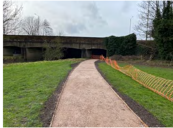
Completed pathway. Source: NWBC
