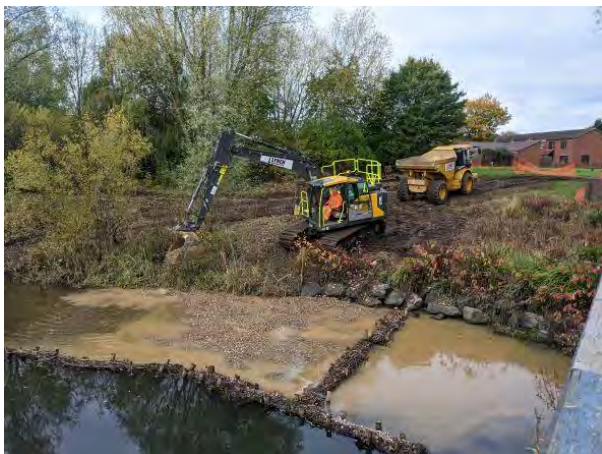
During works, installing natural twig bundles and gravel. Source: Tame Valley Wetlands
