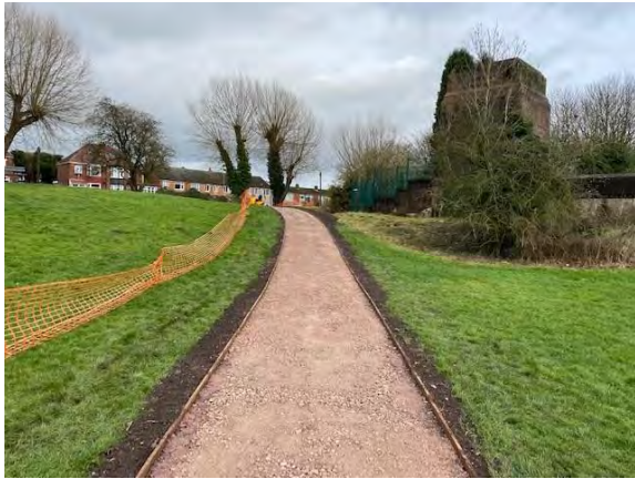
Completed pathway. Source: NWBC
