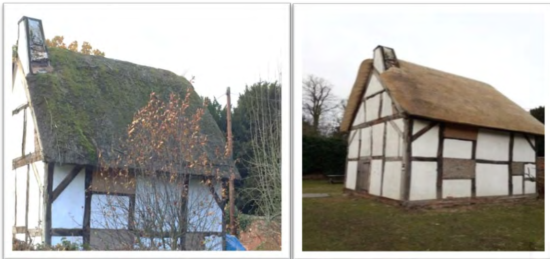
Figure 20: Lea Ford Cottage, before and after replacement of the thatched roof (TVW 2019)
